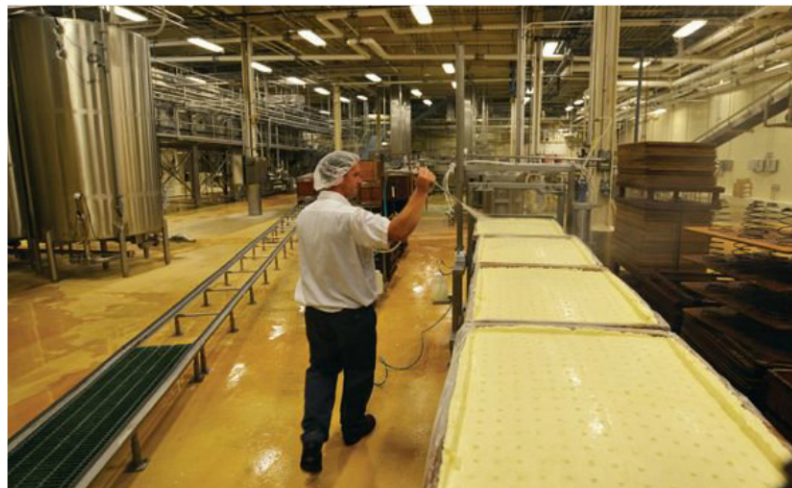
■ A Cheddar room at an Agri-Mark plant. The company has four facilities in Massachusetts, New York and Vermont.
